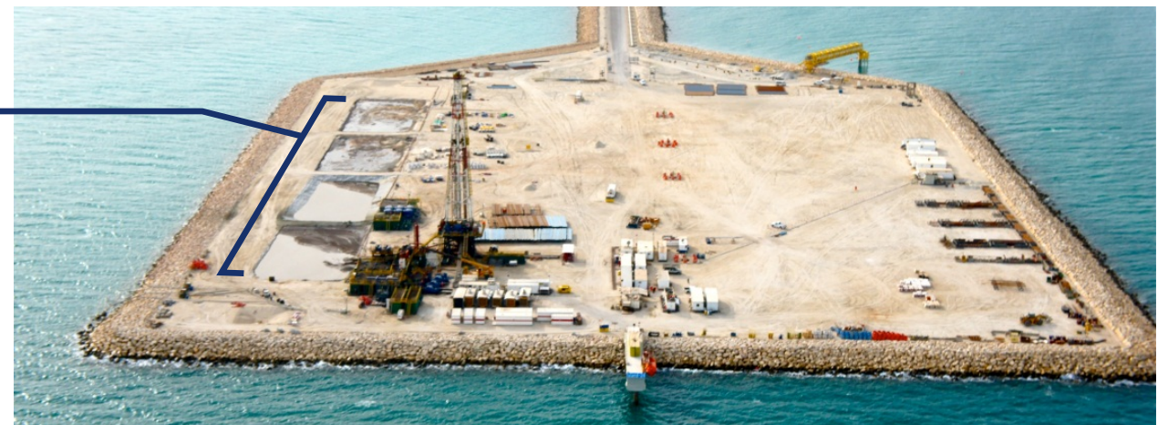
Waste pit at rig site while drilling in normal conditions
