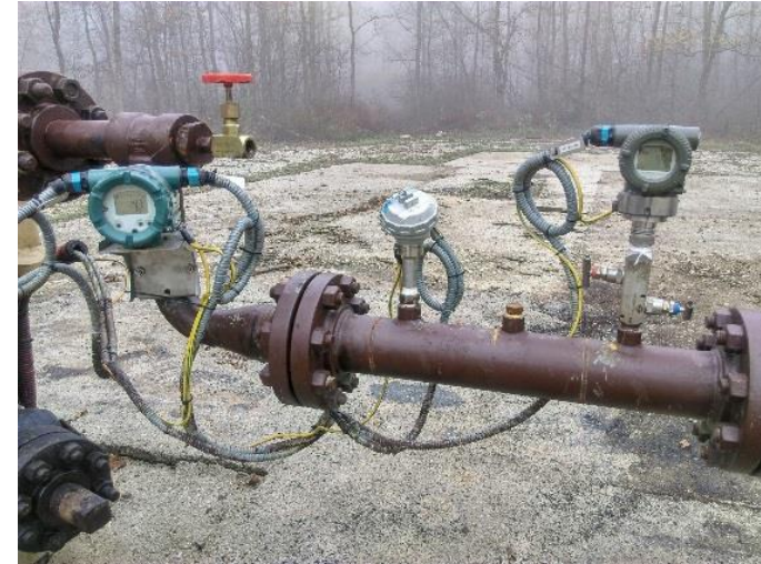
Flowline pressure and temperature transmitter
