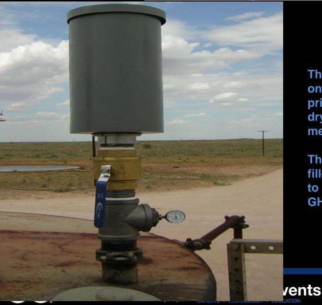
The Bio-Filter works on the absorption principle using a dry, glycol based media.
